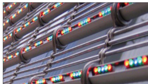
<그림 10> Mediamesh®, woven in steel cables forming a complete façade network 26)
